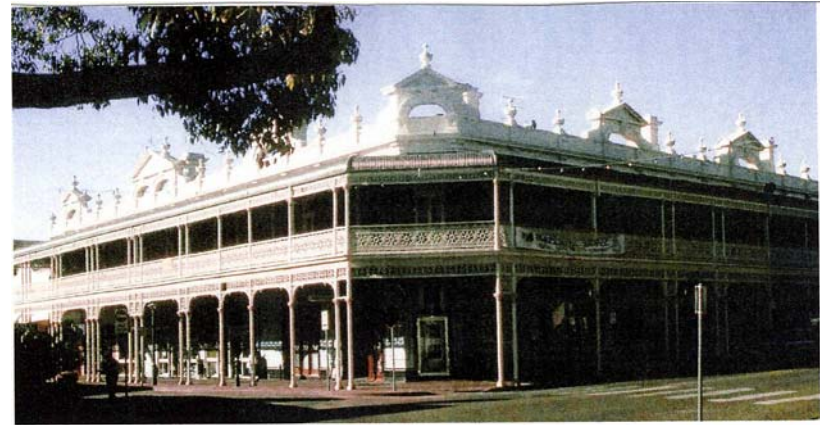
Above: Imperial Hotel, Armidale, J. W. Pender, architect, built c1890 The extensive cast iron balustrades and valances are of Pender’s registered design of 11 May 1885 – used on many of his buildings see ‘Greenwood’, Singleton
