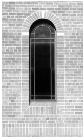
Typical panel and window detail. The motif of key and thrust bricks applies to his many churches.
