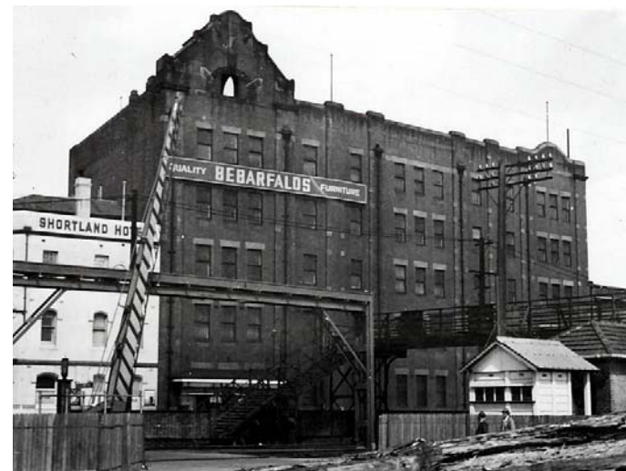
The Warehouse rebuilt, Menkens & Castleden, architects, 1908. Note the corner gable masking a water tank behind. Photograph 1956.
