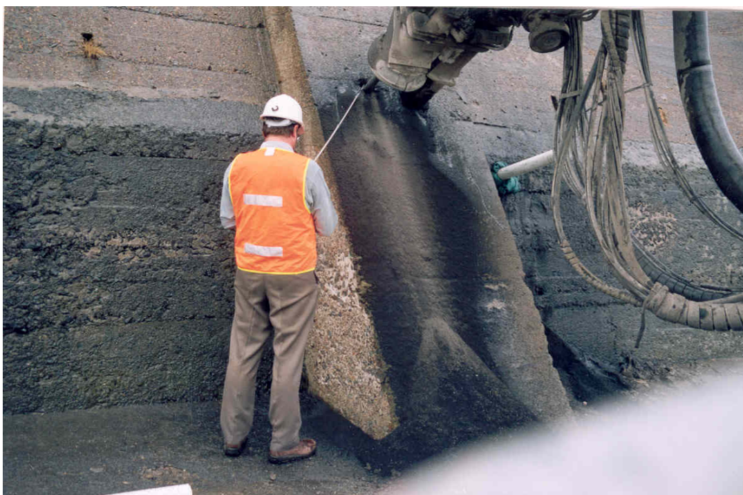
DRIFT 2 – Testing for Explosive Gas in Borehole
