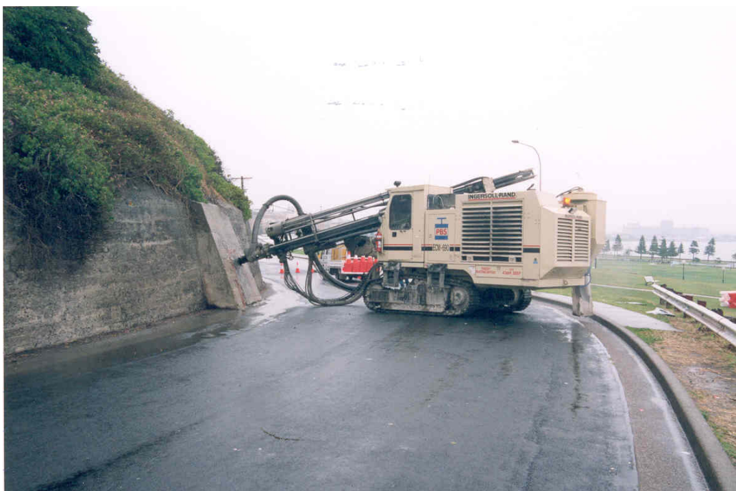
DRIFT 3 – Drilling of Borehole
