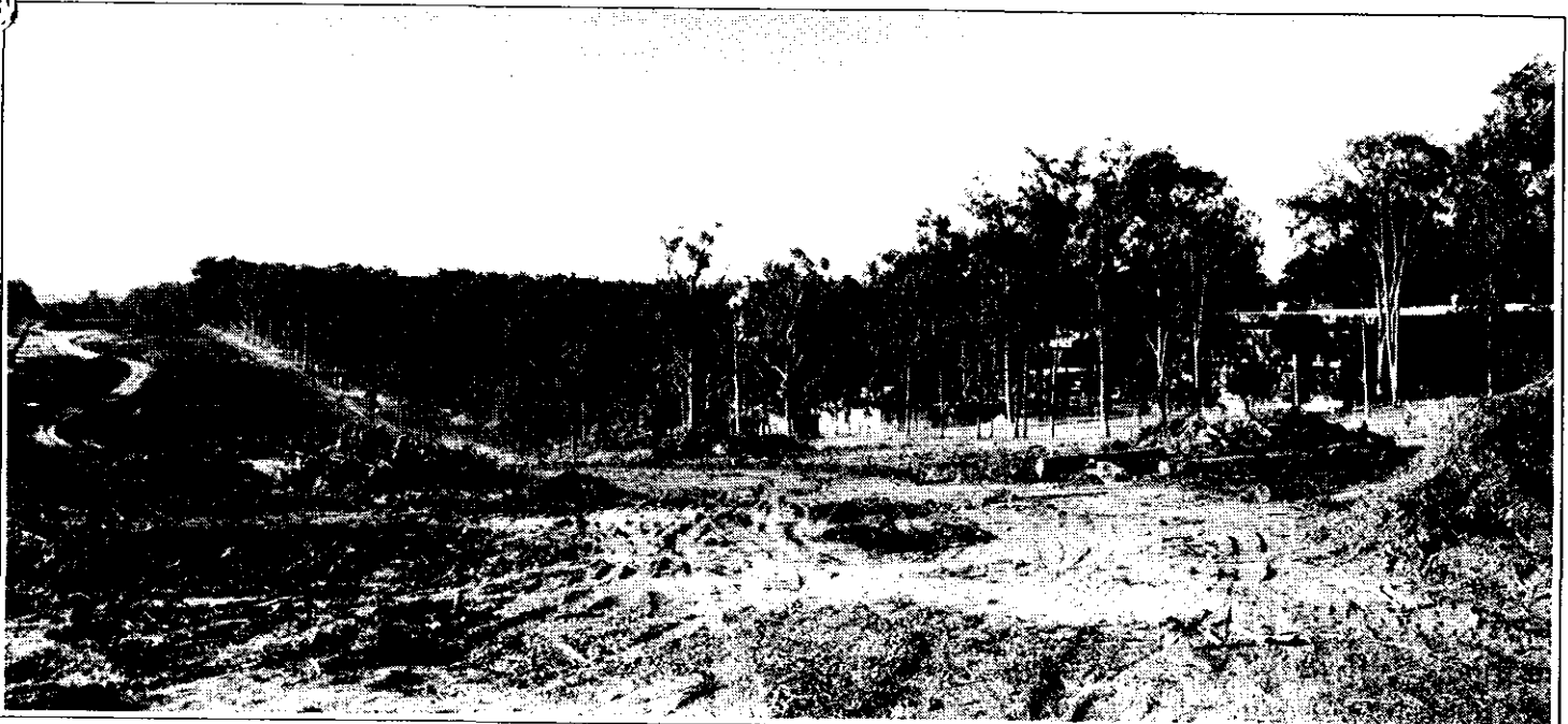
Route cleared for Highway 23
