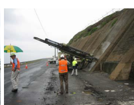
The historic drill into Newcastle's lost convict mine on 26 September 2006. A camera was sent down the drill holes giving Novocastrians their first peek into the 'labyrinth' of Newcastle and Australia's first convict coal mine, first carved out over 200 years ago.
