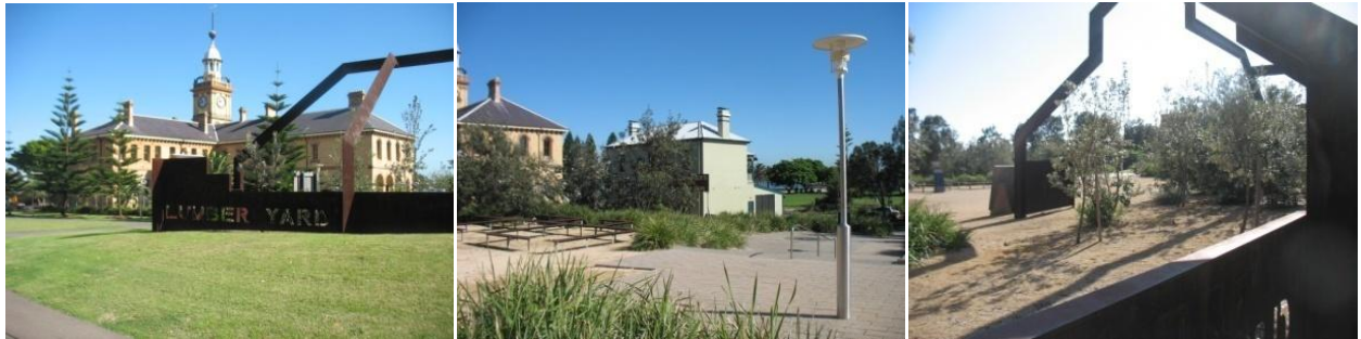
Photograph- Convict Lumber Yard (2008)
