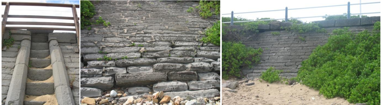
Photograph- Macquarie Pier (2008)
