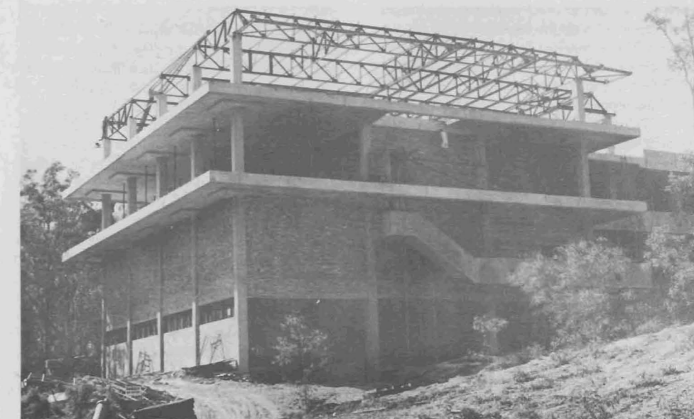
Work on the construction of Stage 11A of the University Library.
